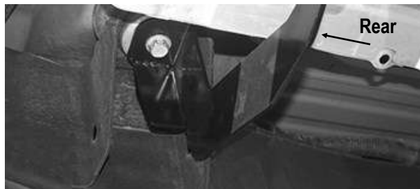
(Fig 9) Passenger Rear Mounting Bracket Installed
