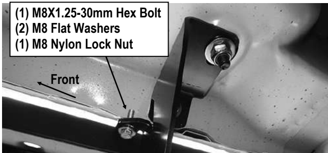
(Fig 17) Passenger 2nd Mounting Bracket Attached to the Pinch Weld
