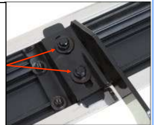
(Fig 17) Step Bar Installed on Bracket Installed (Example)
