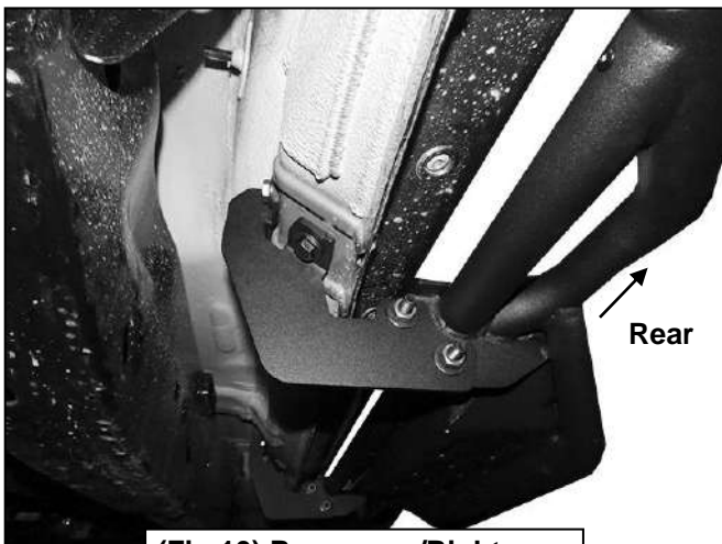
(Fig 10) Passenger/Right Rear Running Board installed
